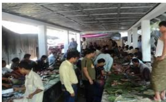
The market-shed constructed by CHTDF
