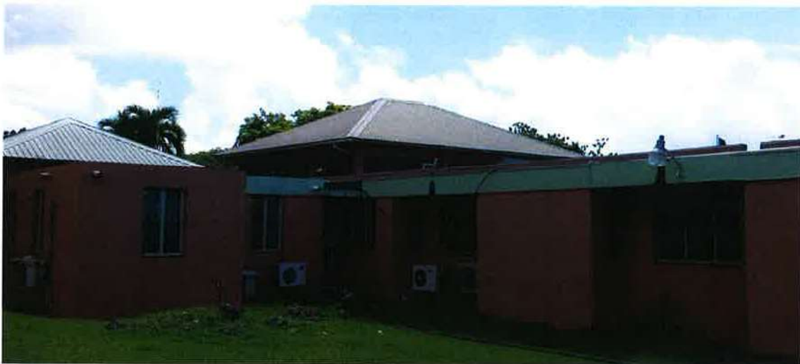
Figure 33: Roof Section - Photograph 1
