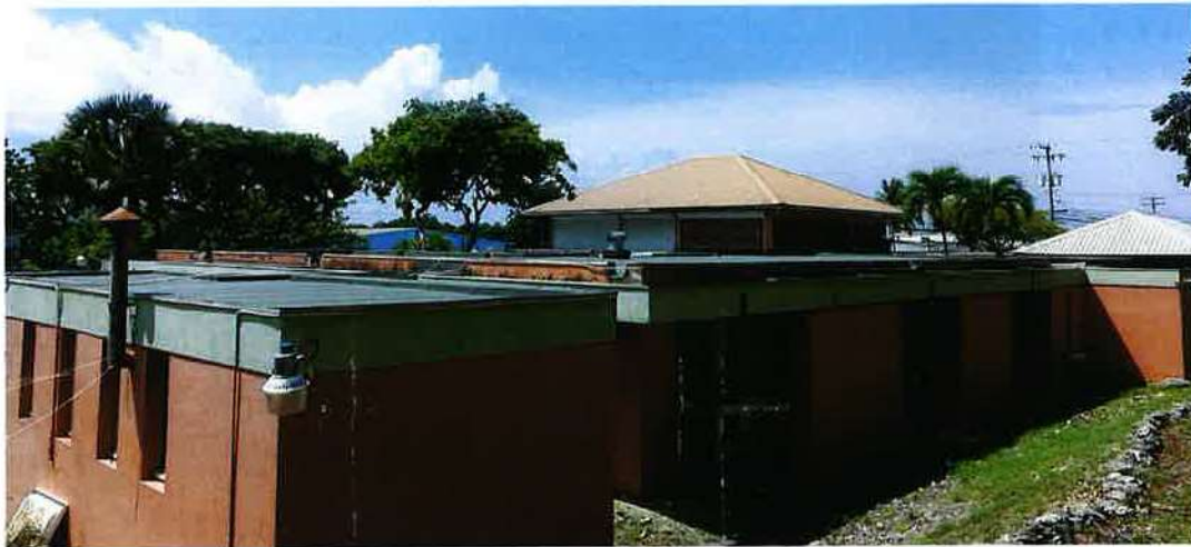
Figure 34: Roof Section - Photograph 2
