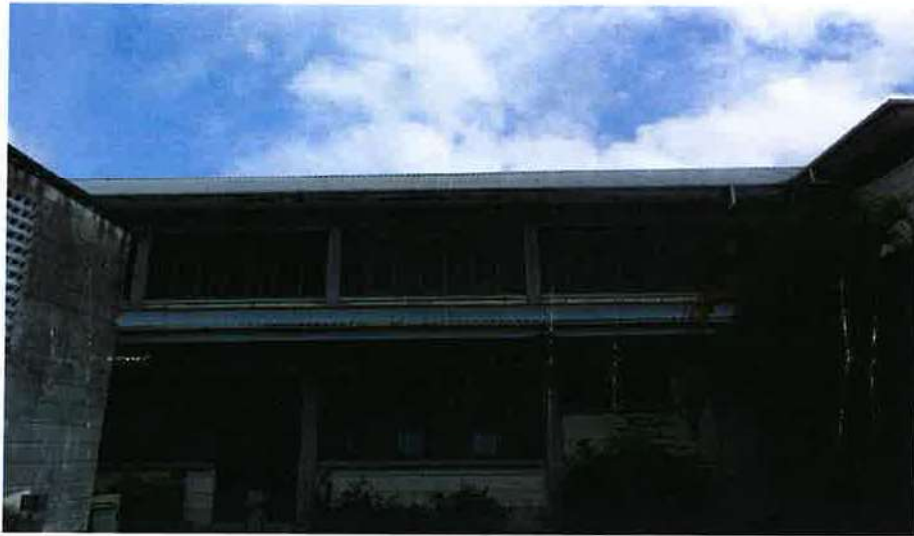
Figure 42: Roof Section - Photograph 3
