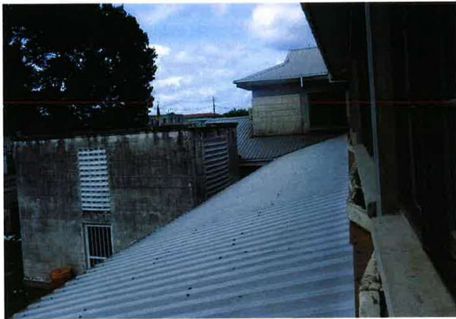
Figure 41: Roof Section - Photograph 2
