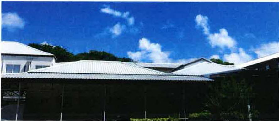
Figure 21: Roof Section – Photograph 3
