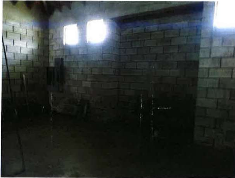
Figure 38: Air conditioning plant room – proposed location for PV equipment
