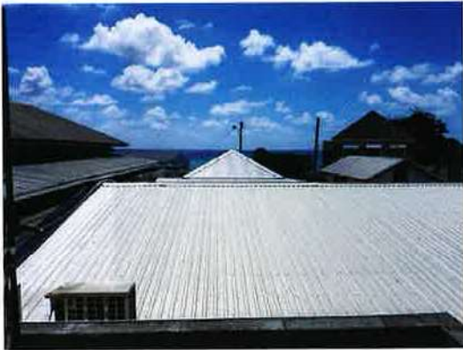
Figure 12: South facing roof section
