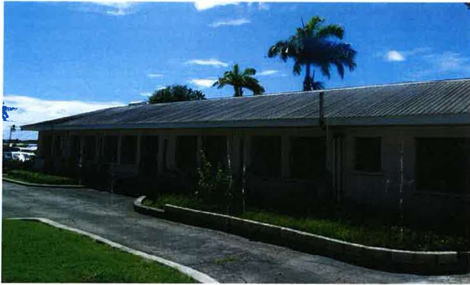
Figure 55: Roof Section - Photograph 1
