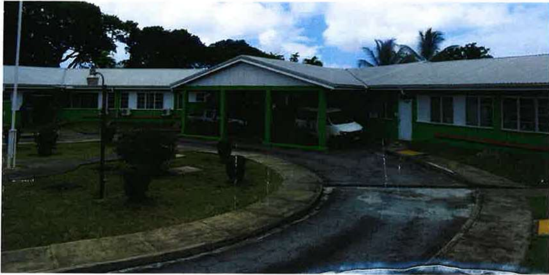
Figure 26: Roof Section - Photograph 1
