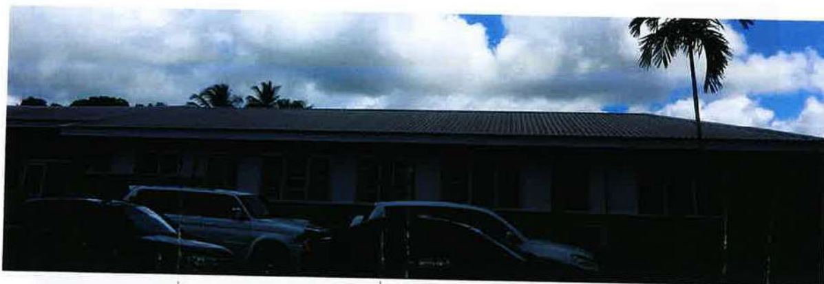
Figure 28: Roof Section - Photograph 3
