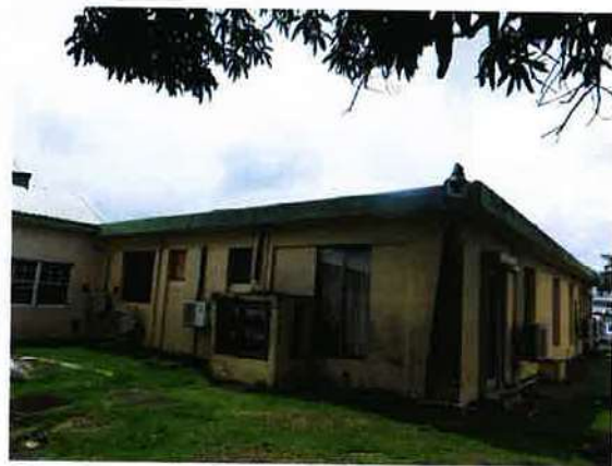
Figure 5: Roof Section Photograph 2
