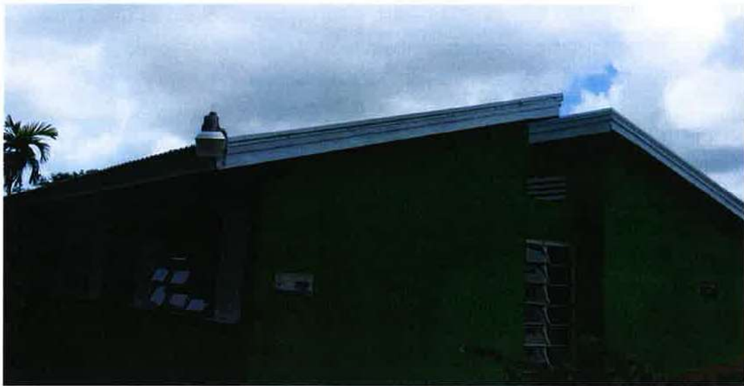
Figure 27: Roof Section - Photograph 2
