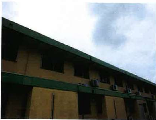
Figure 4: Roof Section Photograph 1
