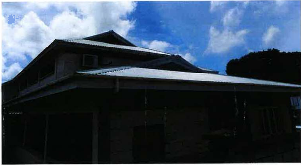
Figure 40: Roof Section - Photograph 1
