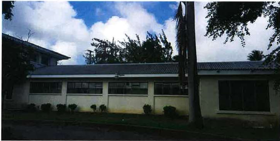
Figure 56: Roof Section - Roof Section
