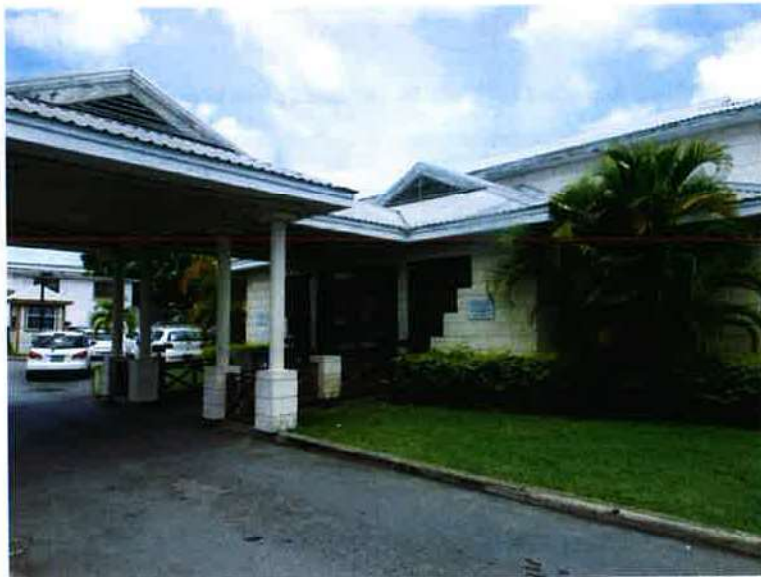
Figure 37: Main Entrance at the Branford Taitt Polyclinic
