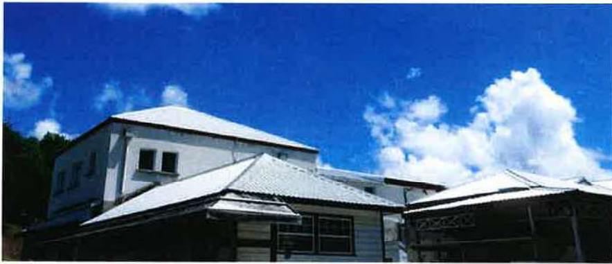
Figure 20: Roof Section - Photograph 2
