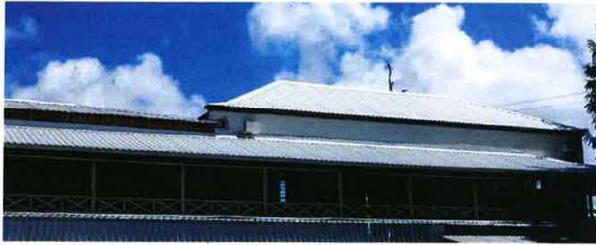
Figure 19: Roof Section – Photograph 1
