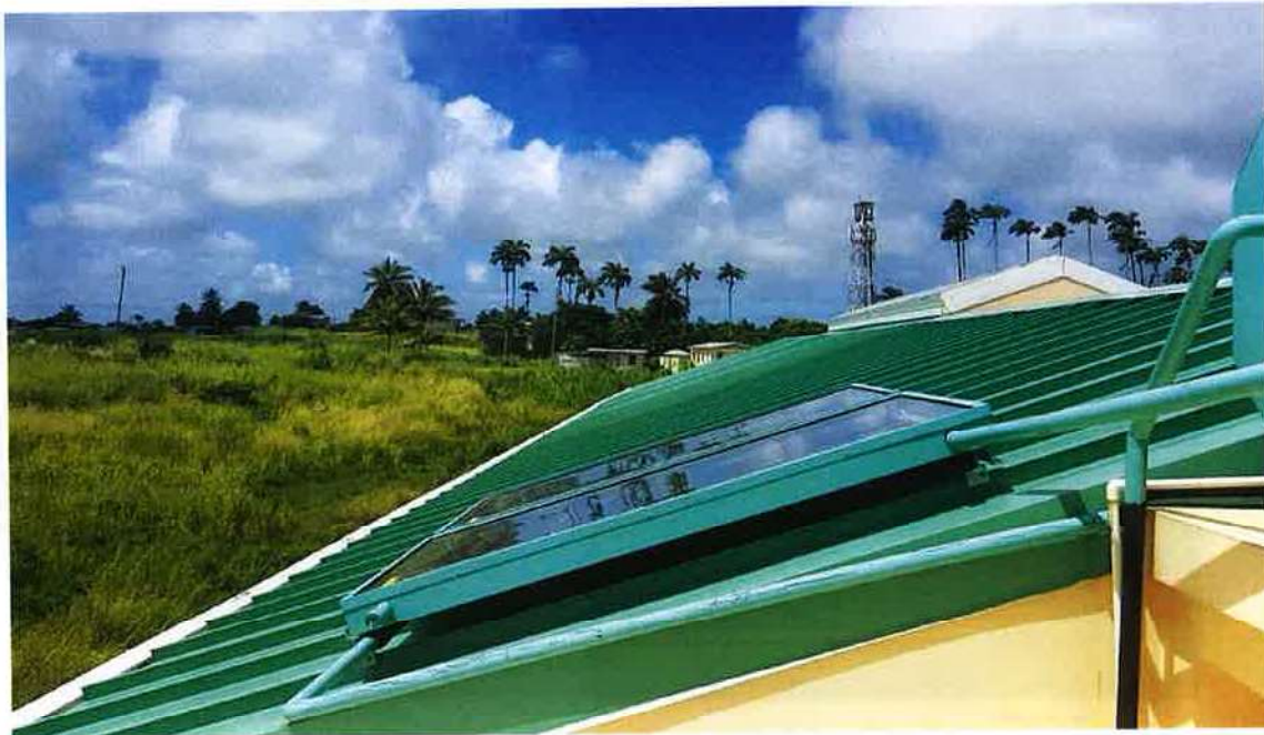
Figure 48: Roof Section - Photograph 1
