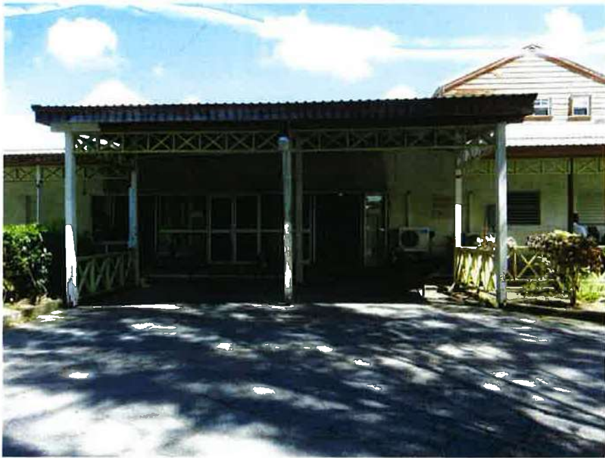
Figure 16: Entrance to Maurice Byer Polyclinic
