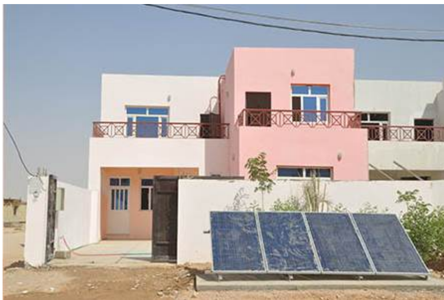
Figure 11. Test solar module installation at the Bytti Complex showing dust accumulation and effects of uneven cleaning.
