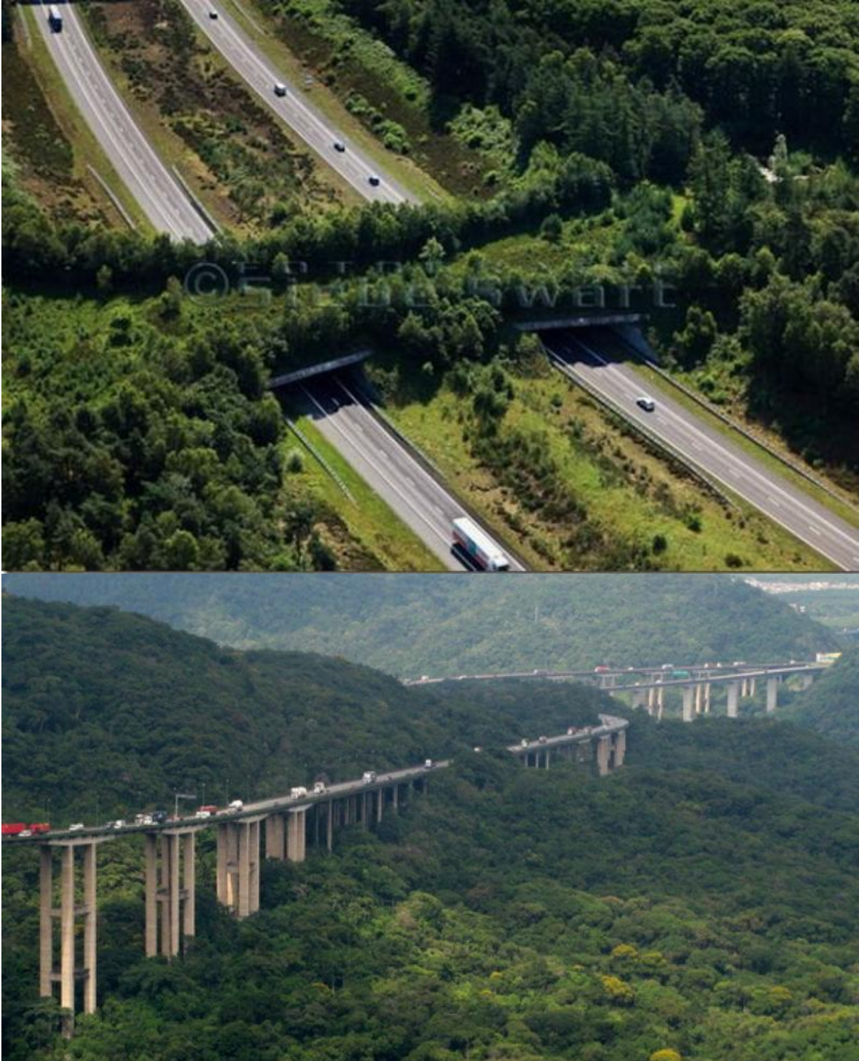
Figure 10. Overpasses and underpasses that allow integration of roads with wildlife crossings. These kinds of infrastructure can be used in planning for Grey and Green infrastructure. Photocredits: top: Ecoduct – Wildlife Bridge – the Netherlands alizul2 blog. Bottom: http://io9.gizmodo.com/5989331/how-well-live-in-a-future-where-cities-have-become-forests
