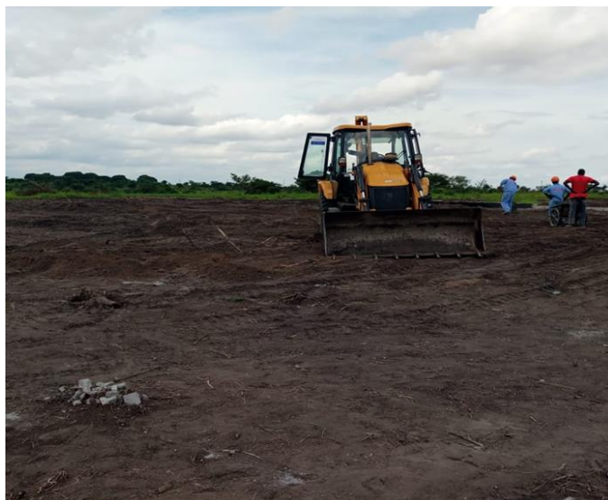
Figure 1: Initial civil works - cleaning the land to prepare construction of the Intermediary Medical Warehouse, Chimoio, Manica province.
