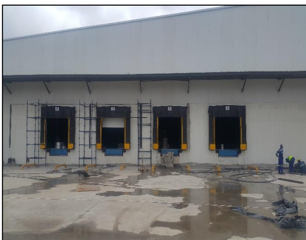
Figures 6 and 7: Image of Zâmbia Medical Warehouse - Dock levelers at Receiving Area (left) and at Dispatch Area – one of UNDP recommendations to MoH Executive Project and that was approved. Will be one of the innovations introduced in Mozambique Medical Warehouses construction Projects.
