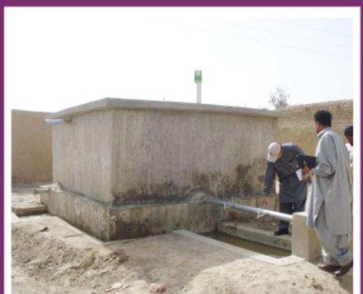
Constructed Water Supply Scheme in Ziarat
