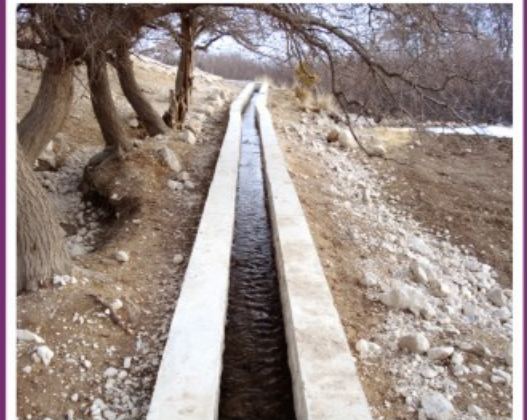
Constructed Water Channel in Killa Saifullah
