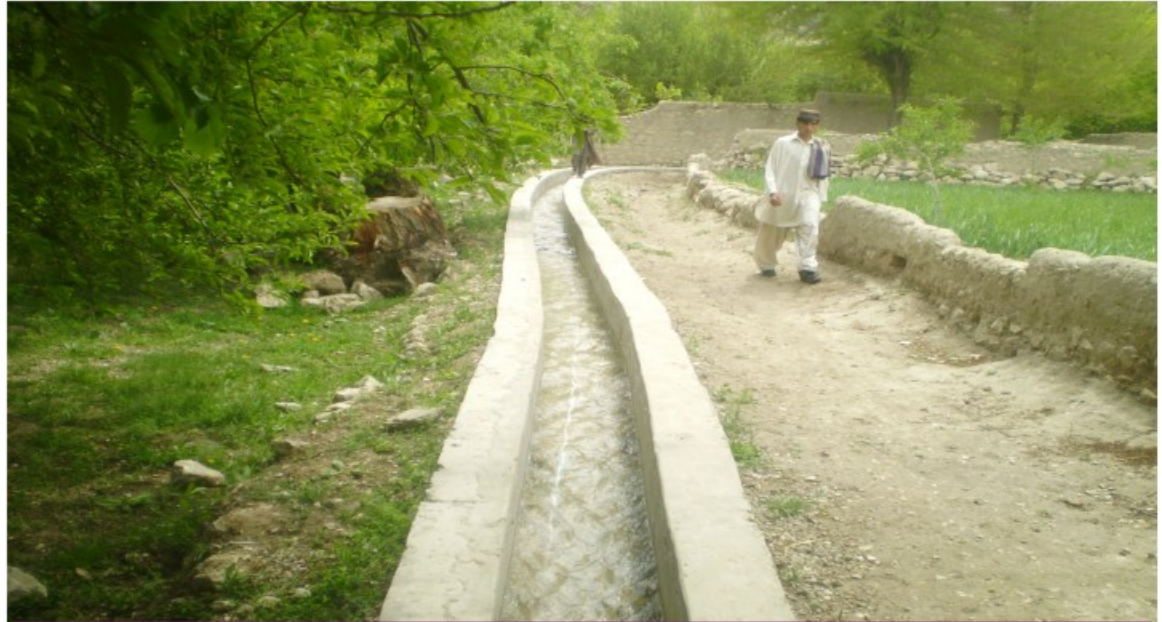
Constructed Water Channel in Ziarat
