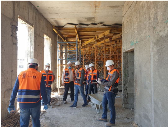
UNDP site team visits the site on 30 April to check the possibility of resuming works
