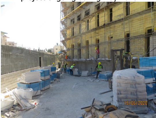
Stone cladding activity started at north façade of Block 1
