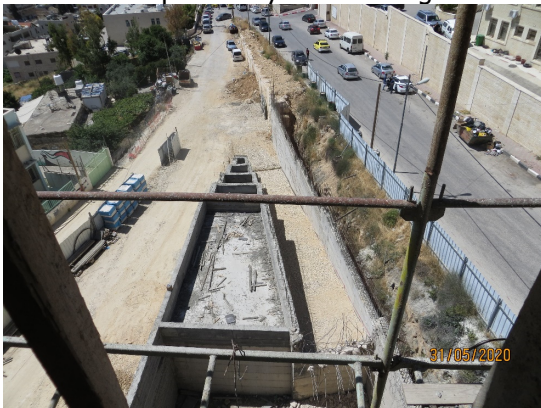
Skeleton works in the Generator and Transformer area at south side of the project ongoing during May 2020
