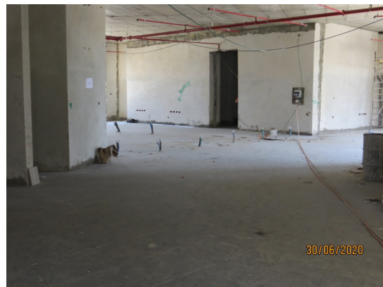
Floor tiling works completed in Ground floor during June 2020
