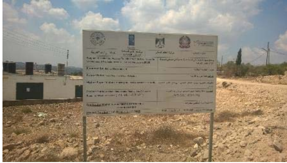
Expansion of connecting roads in Bani Zayed village
