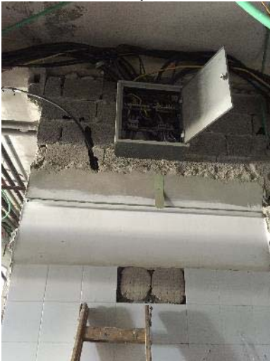
Improvement and rehabilitation of Princess Basmah KG for special education
