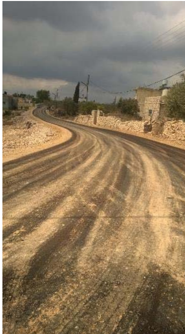
Expansion of connecting roads in Bani Zayed village
