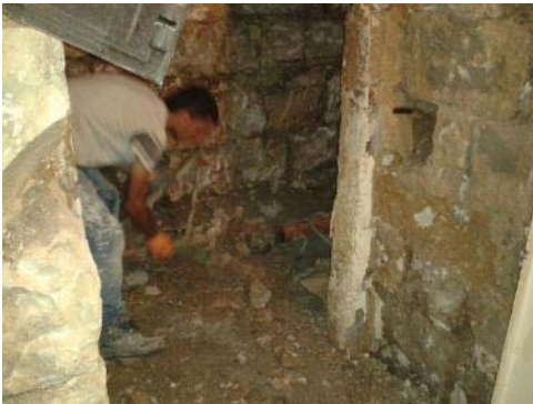
House Rehabilitation in the Old City- Ongoing Rehabilitation
