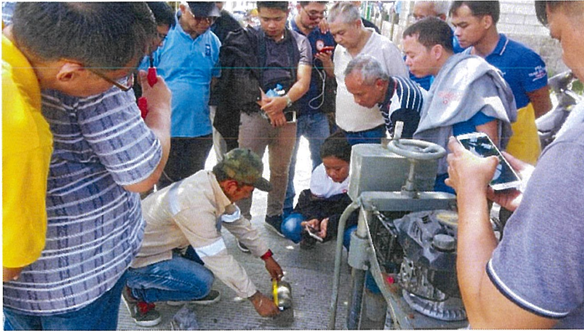
Road Quality Assessment (Coring Test)
