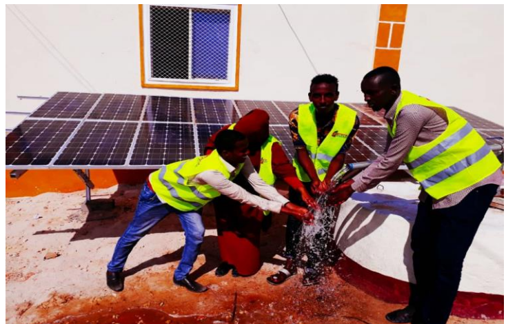
(Fig. 2: Entrepreneurs installing solar water pump in Kismayo)
