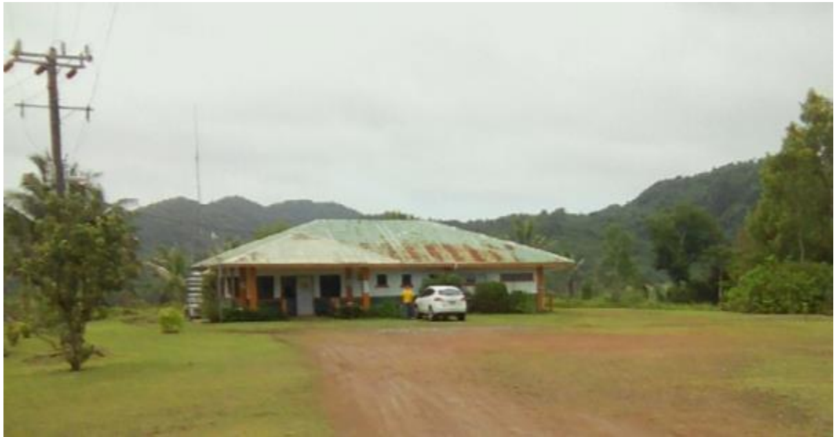
Figure 13 Photo (UNOPS) showing front elevation of WCHC
