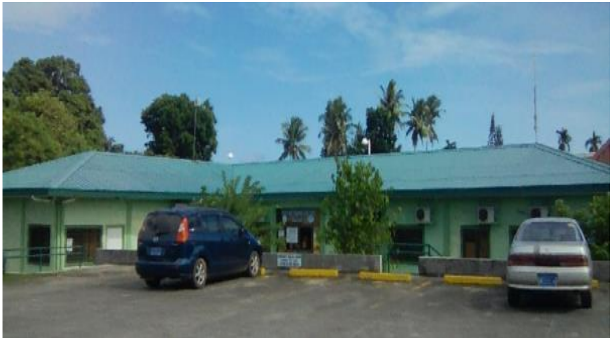
Figure 20 Photo (UNOPS) showing front elevation of CCHCI
