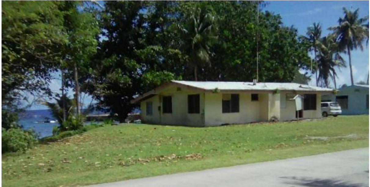
Figure 30 Photo (UNOPS) showing roadside elevation of ACHC
