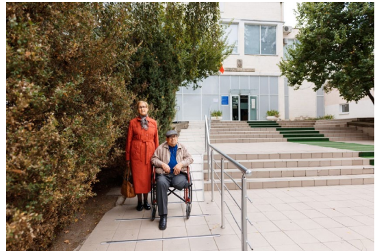
Newly installed access ramp at the local court from Soroca, September 2021.
