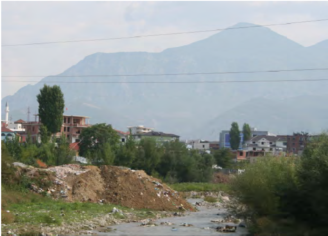
Photo 6: Fill changing flow path of Tirana River
