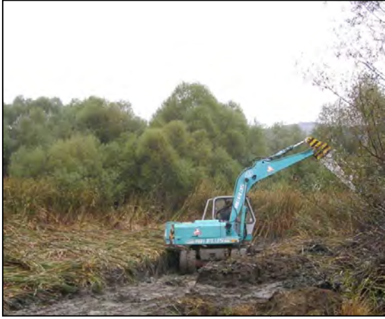
Figure 2: Digging a channel to connect reedbeds with River Rasina
