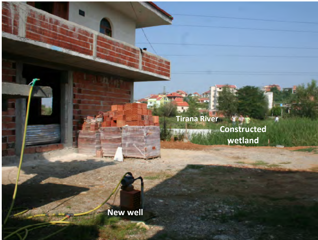
Photo 9: Shallow well in floodplain fill
